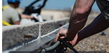
An Airman with the 205th Engineering Installation Squadron from Will Rogers Air National Guard Base in Oklahoma City, secures a half-inch heliax cable to a roof ledge, March 5, 2016, at Tinker Air Force Base, Oklahoma City.
