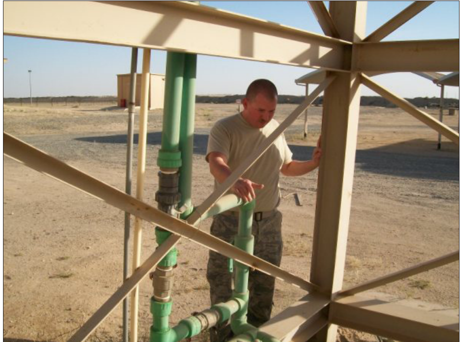
Photo by Master Sgt. Edward Pulver Staff Sgt. Keith Griesel inspects water tank pipes at Ali Al Salem AB, Kuwait.
