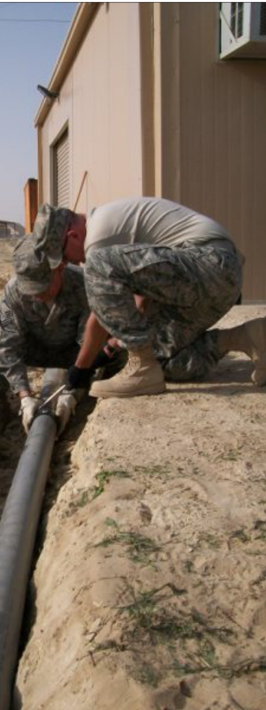
Photo by Master Sgt Edward Pulver Allen Manley replace a sewer line at Ali Al
