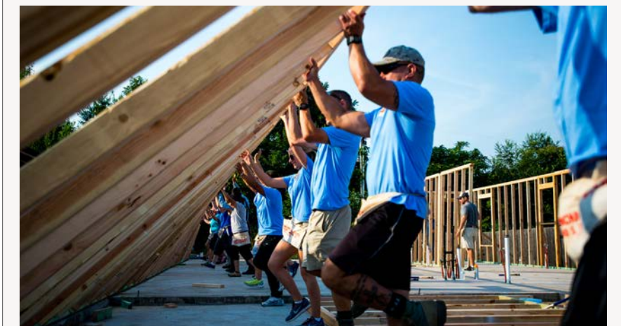
Volunteers from Will Rogers Air National Guard Base work together to raise a frame for a wall of the house. (U.S. Air National Guard photo by Senior Airman Tyler K. Woodward)
