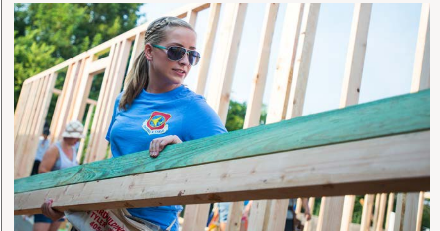
Senior Airman Jessica Morrison, Junior Enlisted Council treasurer, hauls lumber across the construction site. (U.S. Air National Guard photo by Senior Airman Tyler K. Woodward)
